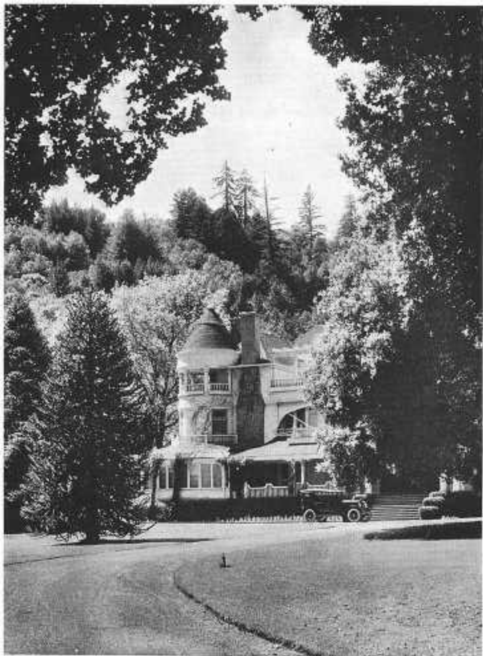
PORTOLA HALL FROM THE MAIN DRIVE
